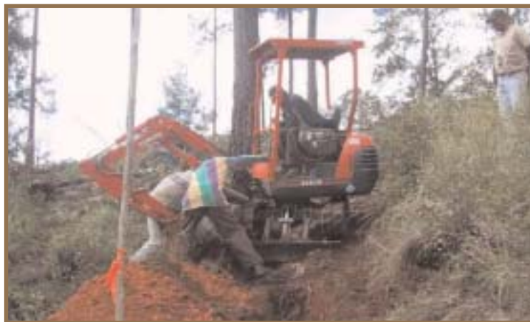
Mechanical trenching on El Corozo Hill
